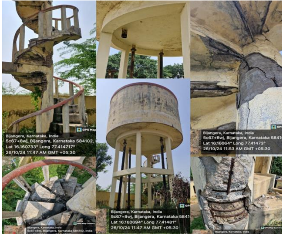
Photograph of Existing Water Tank
