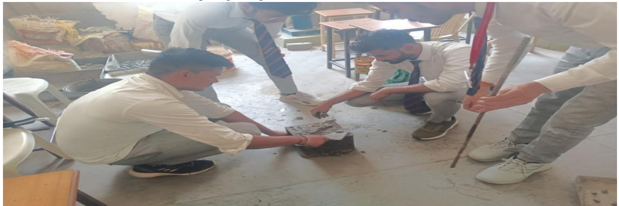
Casting of concrete cubes
