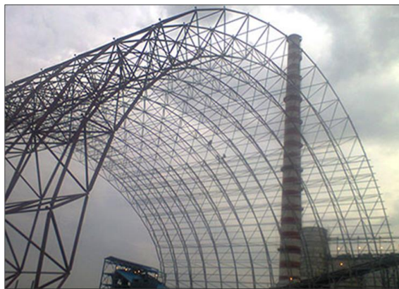
Figure 1.1: Double layer steel braced barrel vault structure
