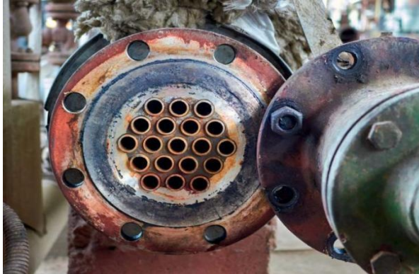
Figure 4.1. Boiler Tube Bundle Open For Maintenance
