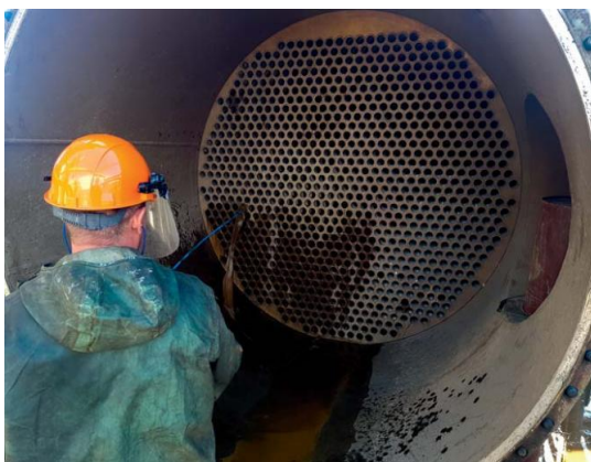
Figure 2.1 Cleaning of Heat Exchanger With High Pressure Hydraulic Unit
