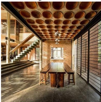
Figure 11. Terracotta pot - filler slab © www.urbannext.net
