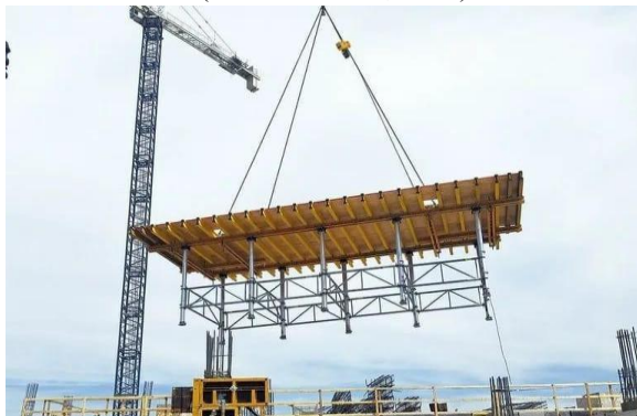
Fig-1 Image representation of a table type of formwork system
