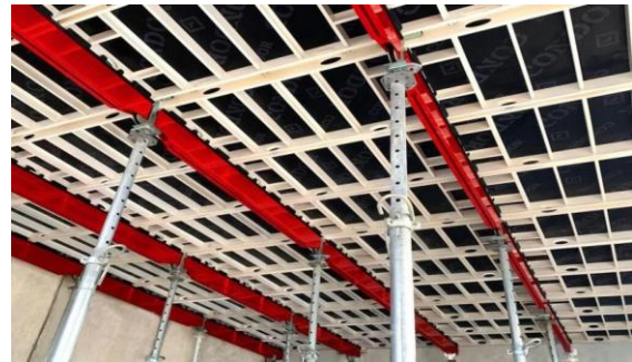
Fig-2 Image representation of a AluDeck type of formwork system
