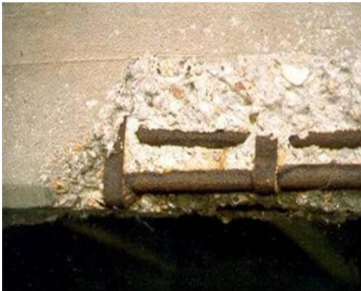
Fig. 2 Carbonation induced corrosion on concrete (Source: corrosion engineering)
