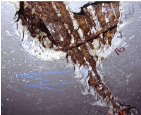
Fig. 3 Chloride induced corrosion on concrete (Source: civil engineering forum)
