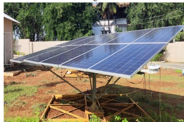
Figure 6: PV Module Mounting Structure
