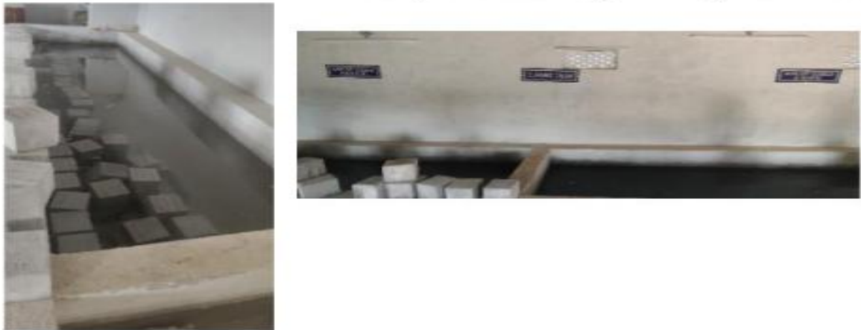
Fig 4. Curing of Casted Cubes
