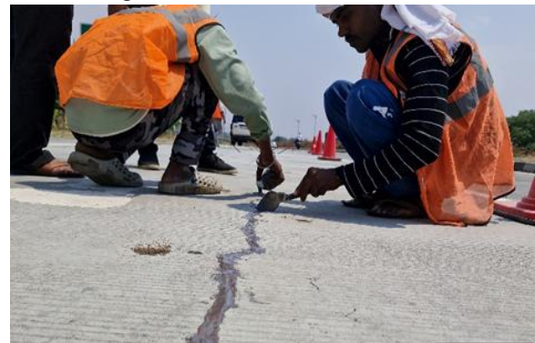
Fig. 3. Sealing of the cracks with Polysulphide base sealants
