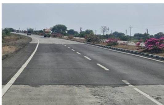
Fig. 4. Over Laying of Bituminous Concrete layer on the PQC
