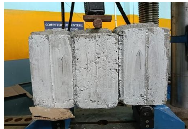
Figure 5. Mode of failure of mortar joint in masonry prism
