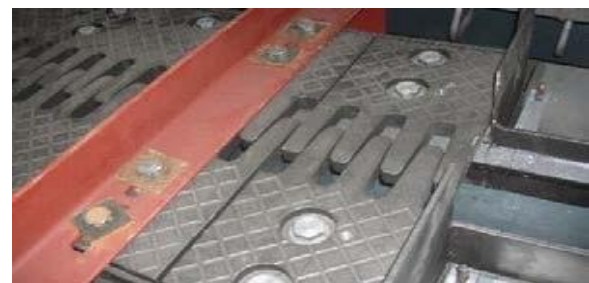
Fig. 4.5. Cantilever (Finger) Expansion Joint with clamping device.
