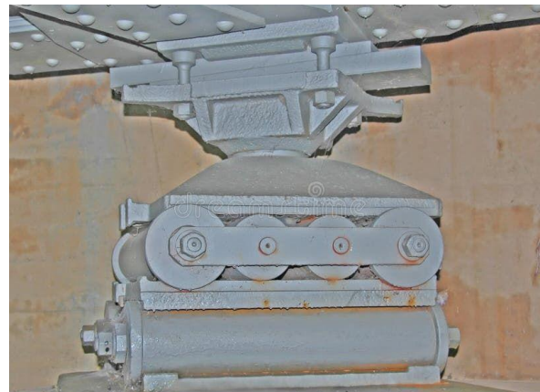
Fig 4 :- Roller Bearing
