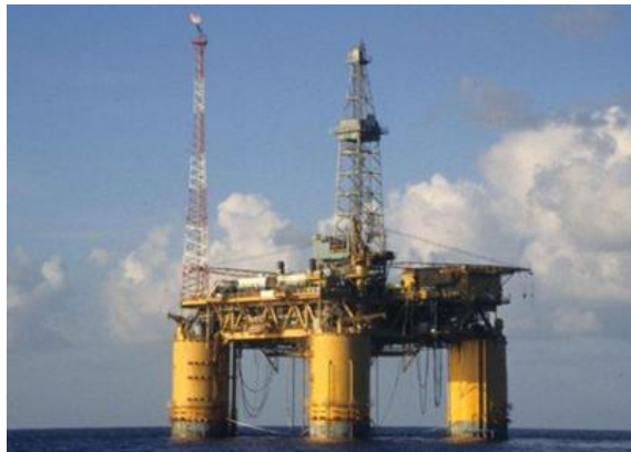
Figure 8: Tension Leg Platforms (TLP) System (Source- Marine insight)
