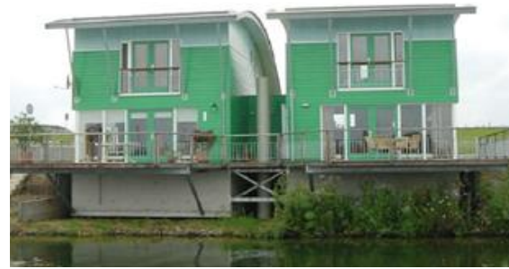
Figure 5: Amphibious floating building (Source- ResearchGate)
