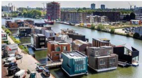
Figure 18: Schoonschip Residential Community (Amsterdam) (Source- Archivibe)
