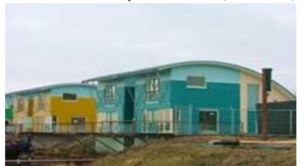
Figure 16: Maasbommel Amphibious Houses (Netherlands) (Source- encrypted-tbn0.gstatic)
