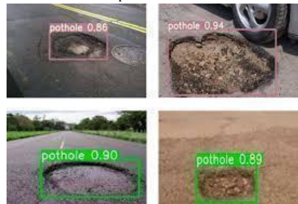
Fig 2. Pothole detection on Roads
