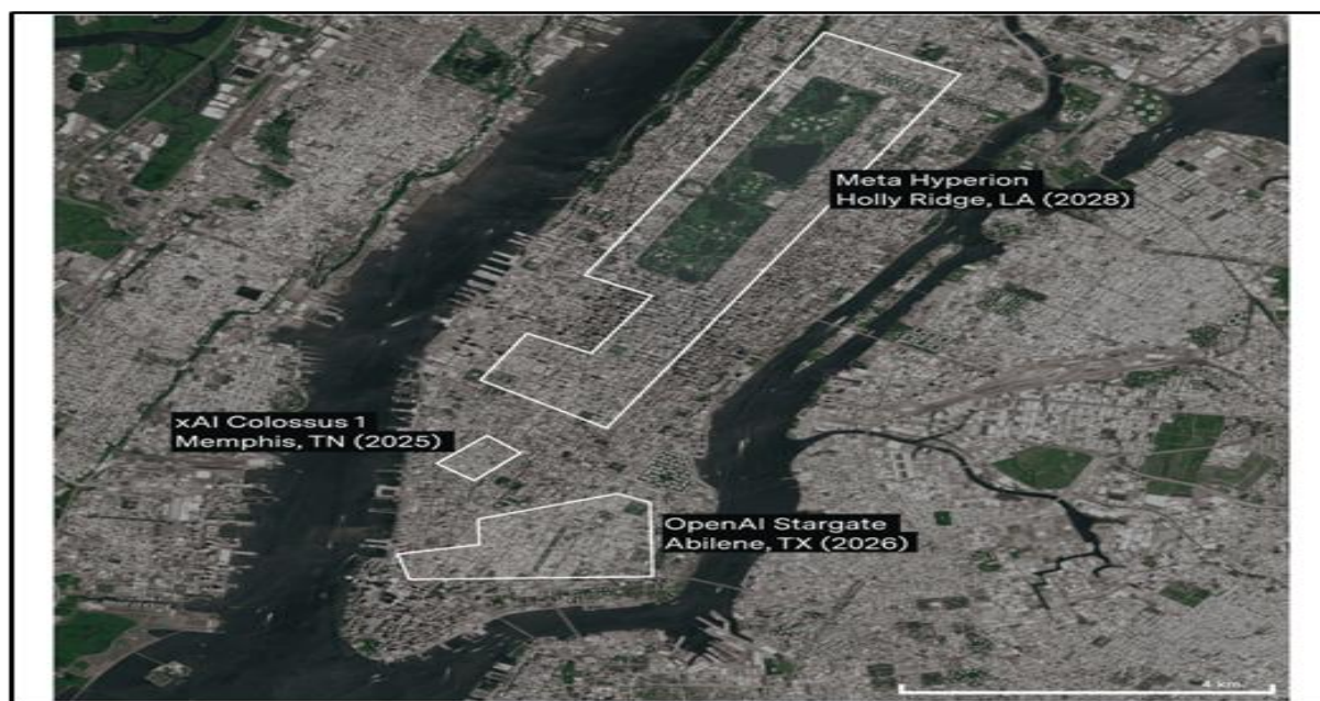
Figure 4: Comparison of the physical size of large hyperscale data center campuses with Manhattan, illustrating the massive land footprint of modern digital infrastructure.
