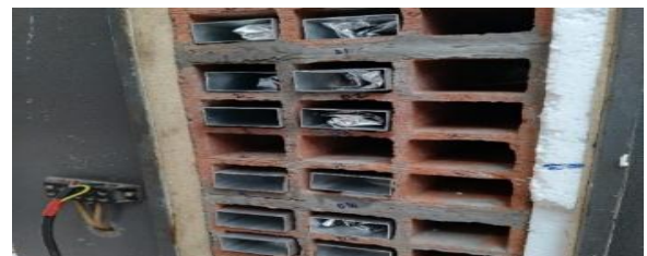
Fig: 18. Porotherm Block with Aluminium Pipe PCM System
