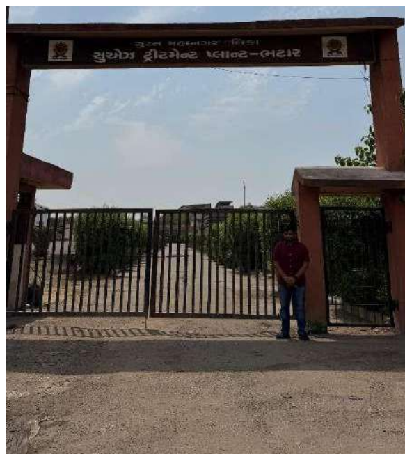
Fig 5.3 Bhatar Sewage Treatment Plant
