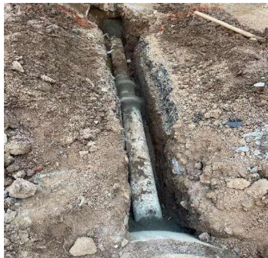
Fig 4.5 Drainage pipe Installation
