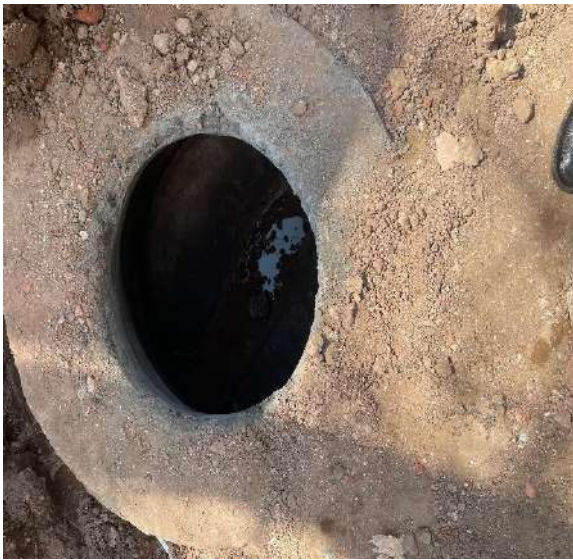
Fig 4.2 Drainage Manhole
