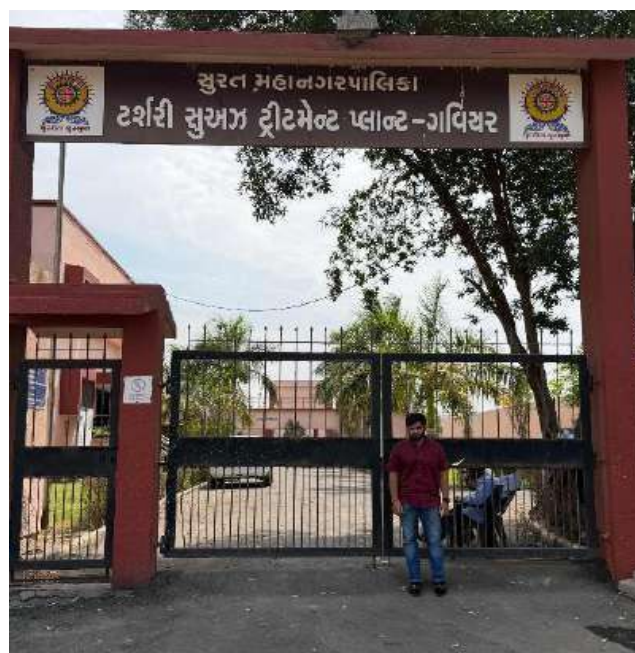
Fig. 5.4 Gavier Sewage Treatment Plant
