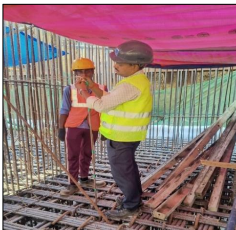
Fig. 4.10.1 • Fixing of Ambient Sensor to Data Logger
