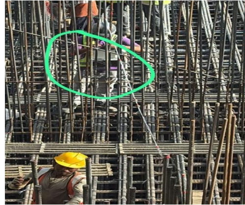
Fig. 4.8.1 • Fixing of Data Logger
