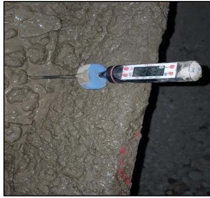
Fig 4.10.3- Concrete Temperature Checking at the time of Pour
