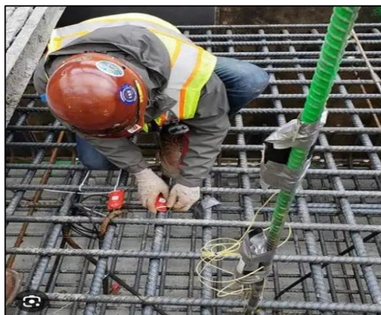
Fig 4.10.2- Installation of Sensor
