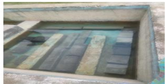
Fig -2: Curing of concrete
