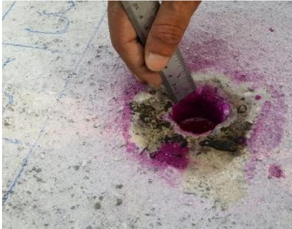
Carbonation Depth Measurement Test
