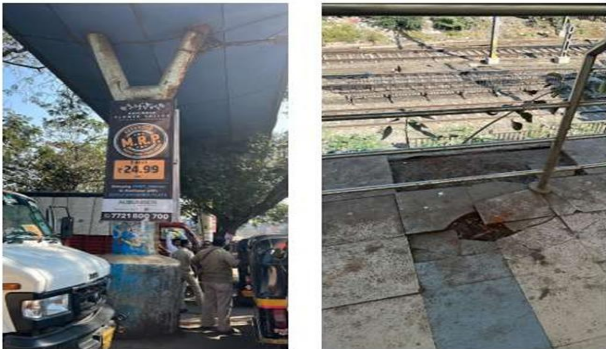
(VIEW OF PIER, DECK SLAB, FLOOR)
