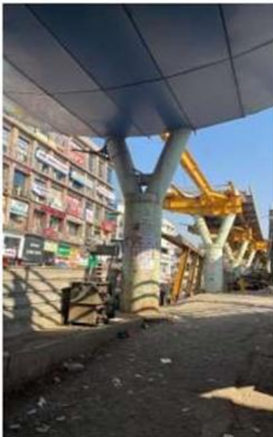
(VIEW OF PIER, DECK SLAB, ROOF)
