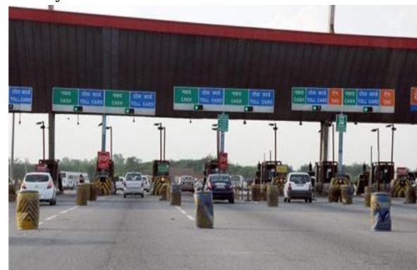
Fig.1. The First Kapsch Toll System in India Finalized
