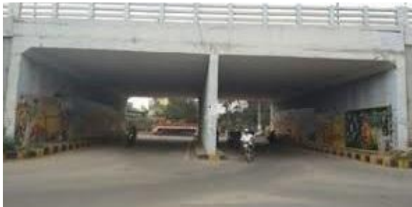
Fig 1.2 VUP & PUP type Underpass (Ref- Highway Correspondence)
