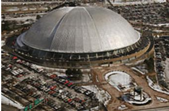
Fig 1 The First Stadium Roof- Civic Arena, Built In 1961
