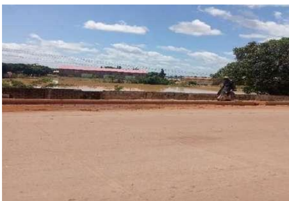
Plate 3: Inundated Buildings along Bye Pass, Kaduna
