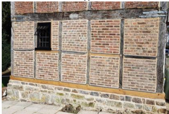
Fig.3.Masonry & Timber Infill Walls
