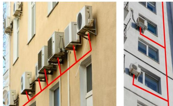
AC Condensed water collection System Image 2
