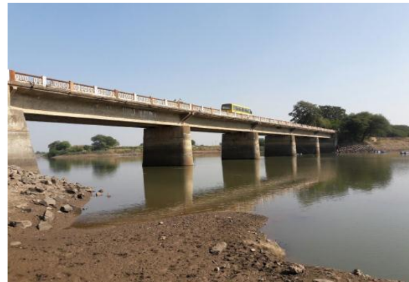
Figure 1. Field view of the Ozar Bridge selected for the SHM case study.
