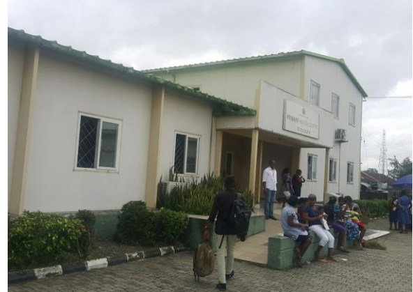
Plate 1: Image of storey building with modular construction.
