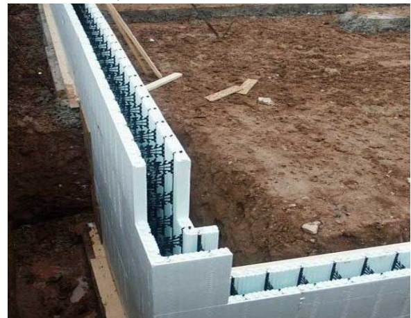
Plate 2: Image of a Concrete Insulated Forms in building construction
