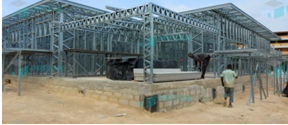
Plate 7: Image of Light-Gauge Steel Framing for building construction
